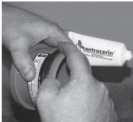
Figure 15: Applying Lubricant to Gasket
