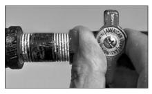
Figure 37 - Manual Gas Valve in OFF position.
