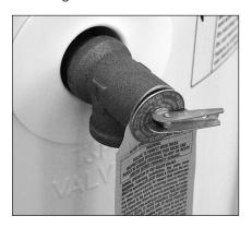
Figure 16 - Temperature and Pressure Relief Valve
