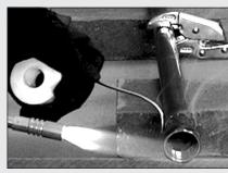
Solder a short length of pipe (about a foot) to a threaded adapter using only 95/5 tin-antimony or equivalent solder. Attach the threaded adapters to the water heater's connections (using thread sealant tape or pipe joint compound). Connect the home's water pipes by soldering, keeping the connections at the water heater cool with wet rags.
