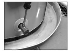
$\label{eq:Figure 31 - Draining the water heater.}$
