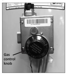
Figure 9 - Turn gas control/temperature knob OFF.
