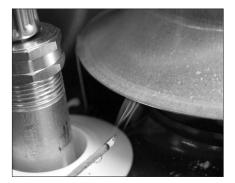
Figure 26 - Test the air supply and vent to make sure the water heater has adequate air and is venting properly.
