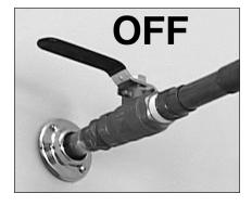
Figure 11 - Cold water supply in OFF position.
